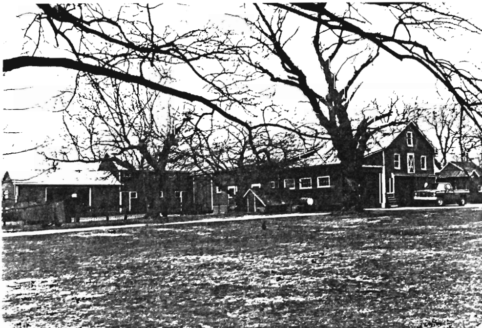
Barn (B) and adjoining sheds
